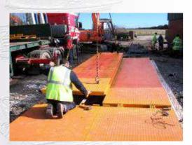
35.3 metre by 3 metre 120 tonne Weighbridge - with indicator and standard ticket printer
